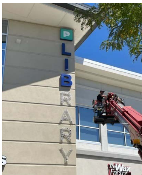
New exterior sign installation at Council Tree
